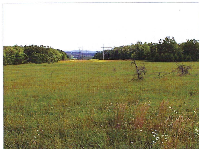
High voltage powerline and ROW, Fairfax Stone, Tucker County, WV.
